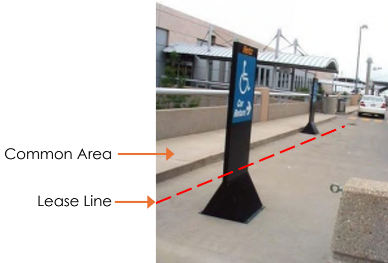
Upper level lease area and curb condition
