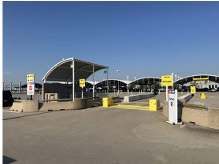
Upper level return entry lane
