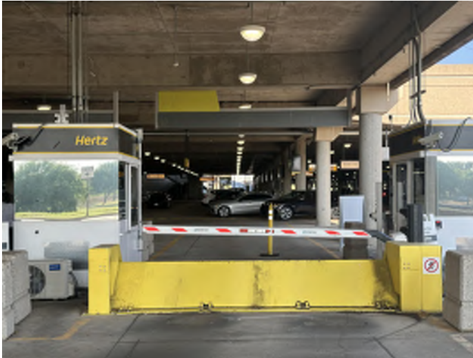
Lower level exit and kiosk
