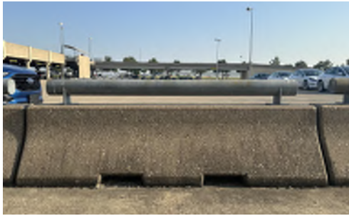
Eight-foot concrete barricade
