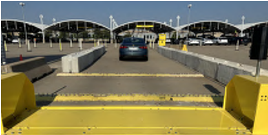
Upper level entry control system
